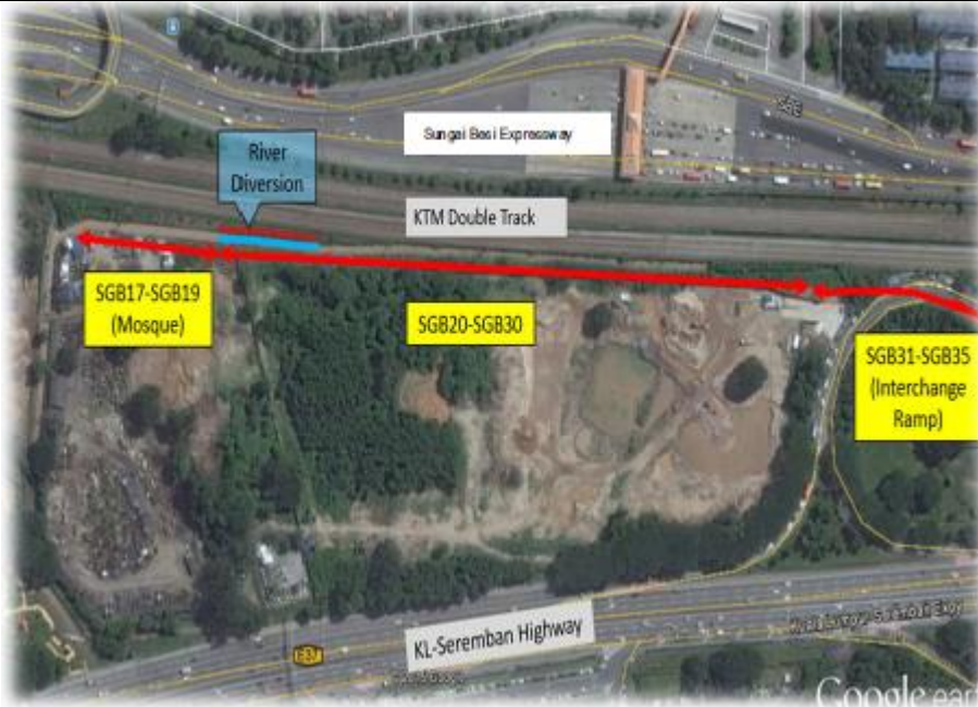
Figure #2 Work area for the recent MRT2 contract
